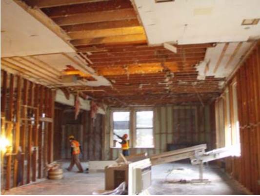
Ceiling Demo Upper Floor North Hall
