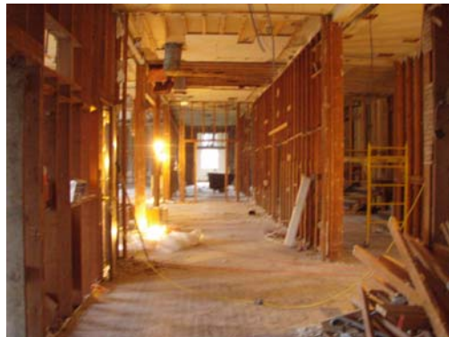
Upper Floor of North Hall
