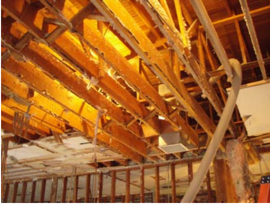
Insulation Removal Upper Floor North Hall
