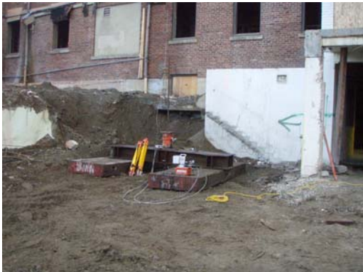
Sacrificial Micropile Test Rig
