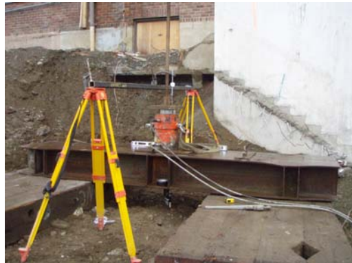
Micropile Tension Test in Progress
