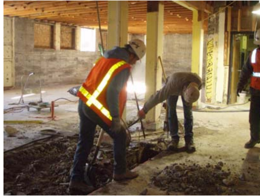
Excavation of Existing Footings at South Hall
