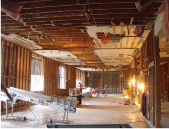
Demo Debris Clean Up North Hall
