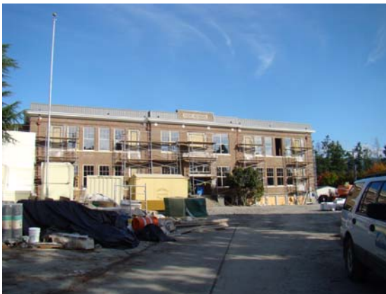
New Windows, Parapet, and Stucco N. Hall
