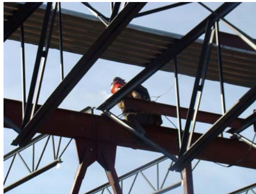
Welding Trusses at Commons
