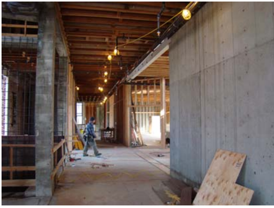
Interior Framing Main Floor S. Hall
