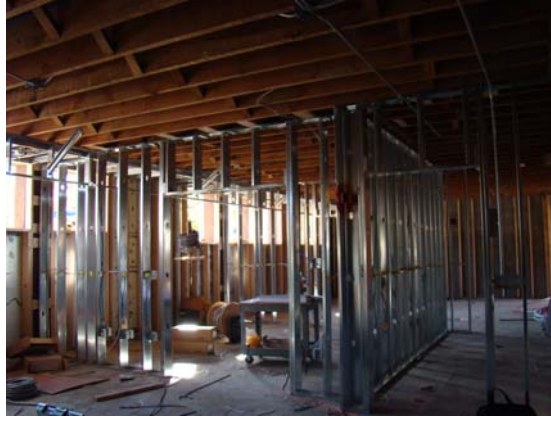
Light Gauge Steel Framing Lower Floor S. Hall
