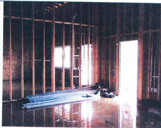
New classroom interior framing, 3-27-09.
