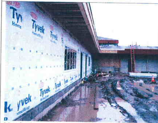
North elevation of addition, 4-1-09.
