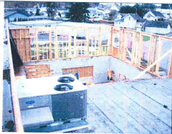
View southwest of music room (high ceiling area), 4-10-09.
