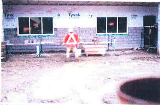
Masonry veneer in progress at south elevation, 4-1-09.
