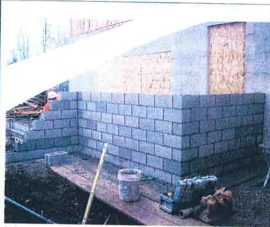
Masonry wall south of Music room, 4-10-09.
