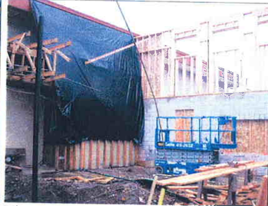
View looking southeast from inside music room, 4-10-09.
