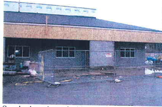
South elevation of addition, 4-10-09.
