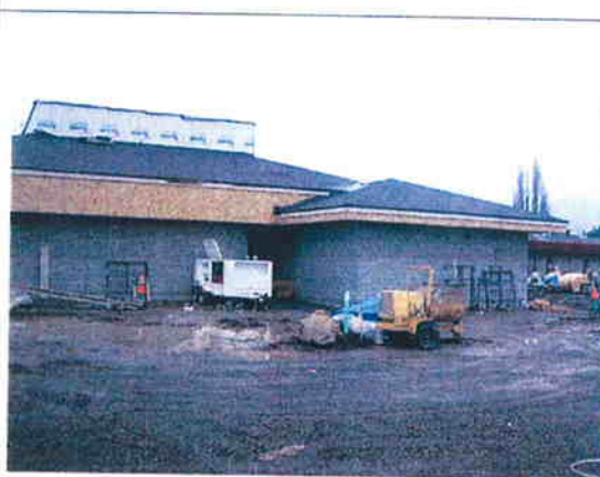
East elevation of addition, 4-10-09.
