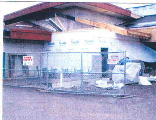
Southeast corner at kitchen/multipurpose, with masonry veneer and building wrap, 4-10-09.
