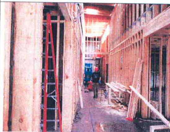
East/west corridor at addition, 3-27-09.
