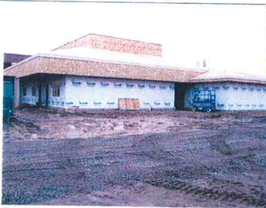
East elevation of addition – ready for roofing and masonry veneer, 3-27-09.
