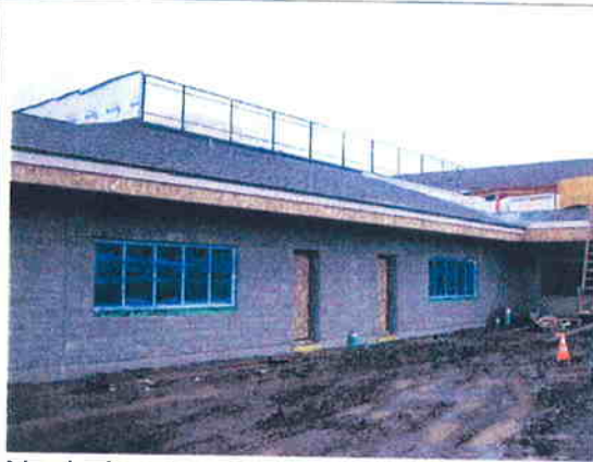
North elevation of addition, 4-10-09.
