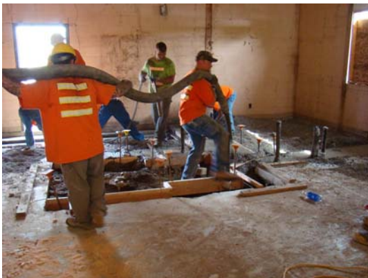
Pouring New Footings at Locker Rooms
