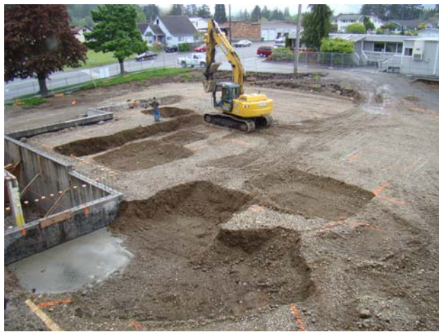
More Footing Excavations for New Commons
