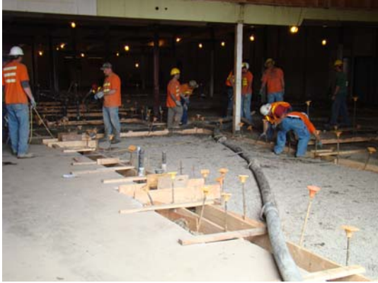
More New Footings at Locker Rooms
