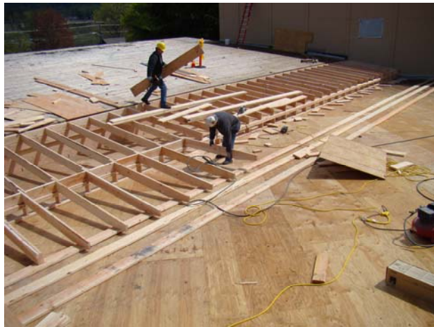
New Roof Overbuild at Locker Rooms
