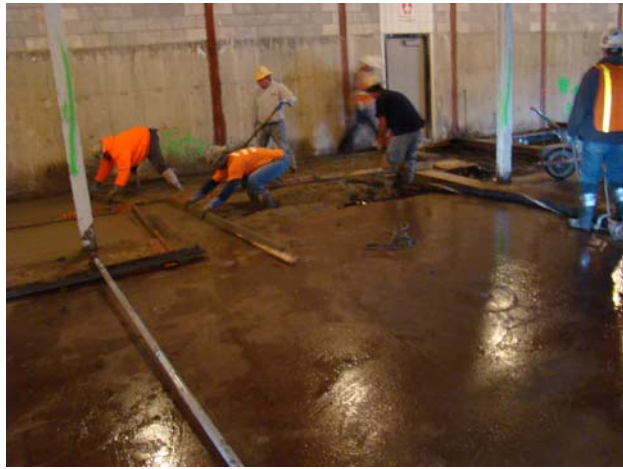
New Concrete Slab at Locker Rooms
