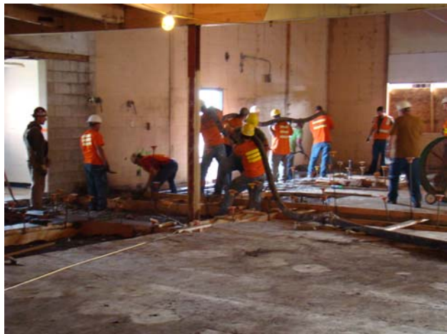
Pouring New Footings at Locker Rooms
