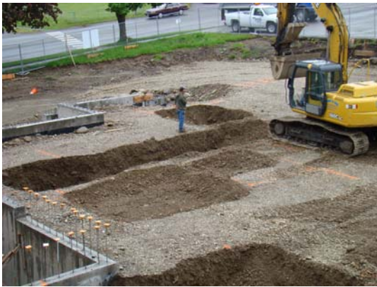
Footing Excavation for New Commons
