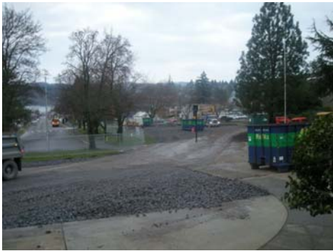
Erosion Control Placement
