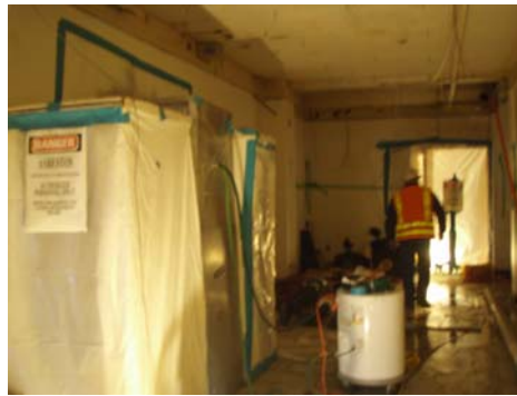
Asbestos Abatement in Kitchen
