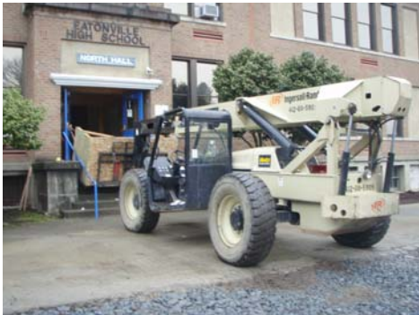
Demo Debris Removal North Hall
